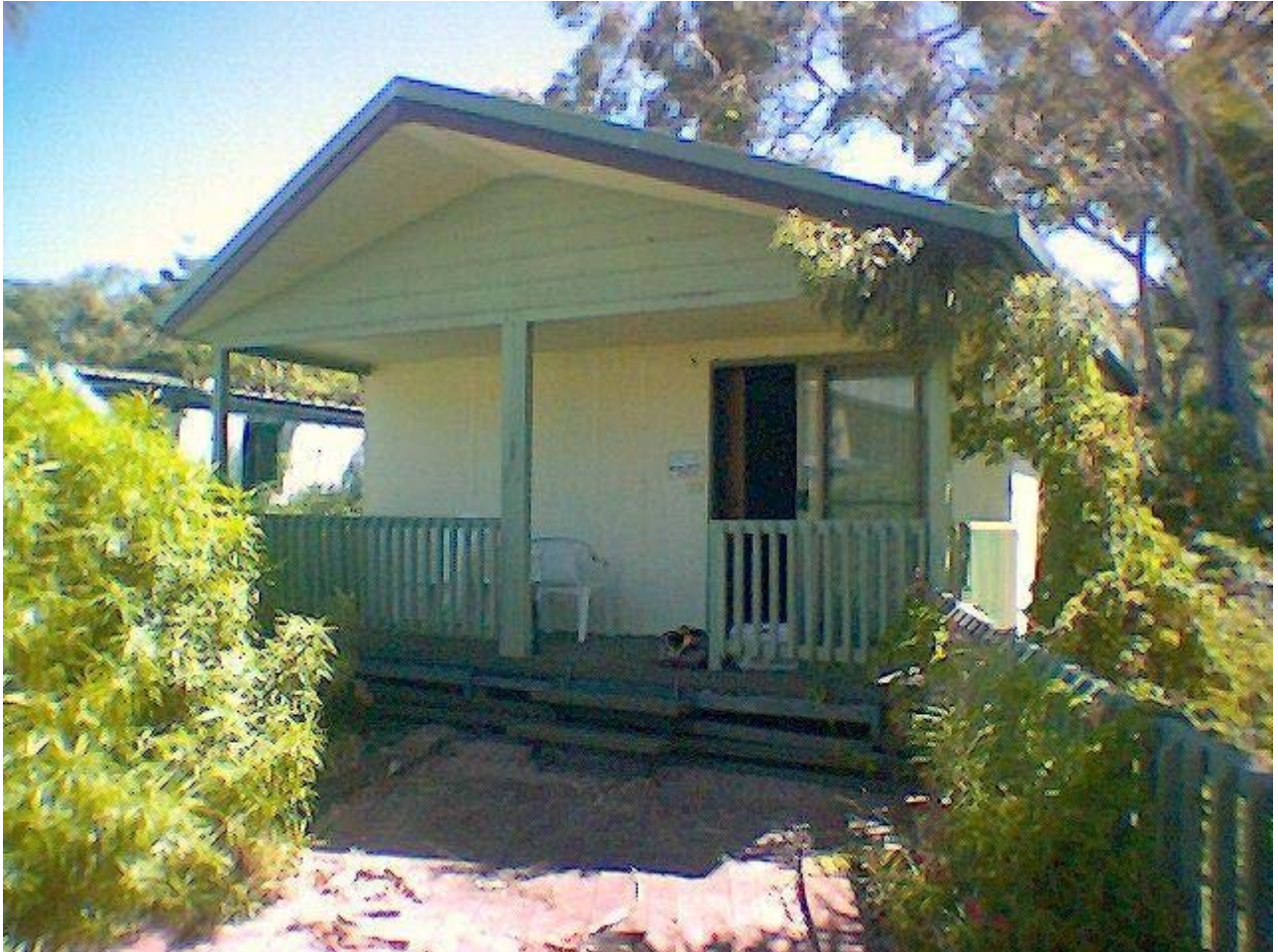
Spa/Sauna Quoin Island
